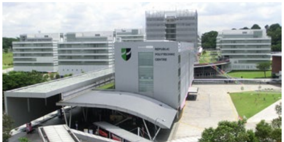
Republic Polytechnic Center, Singapur, 2006
