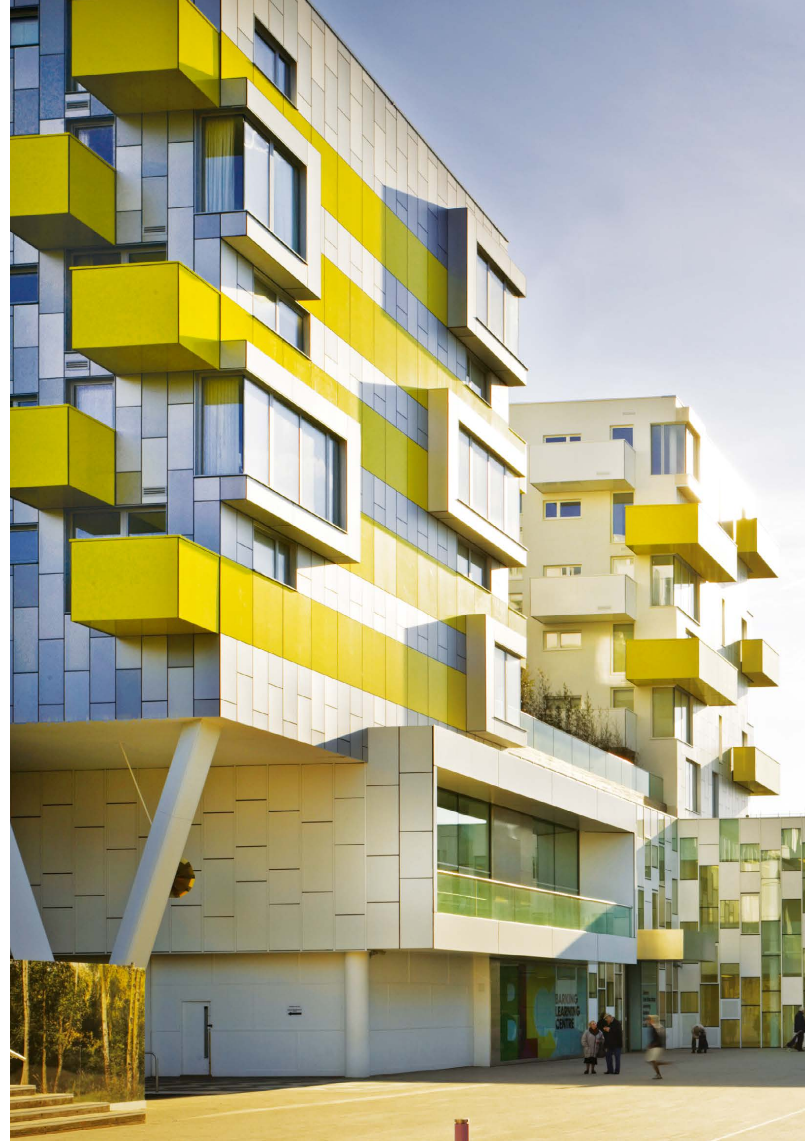
RIGHT, Project 148: Lifelong Learning Centre Barking Project Participants Architect: Allford Hall Monaghan Morris Facade: Cladding UK
