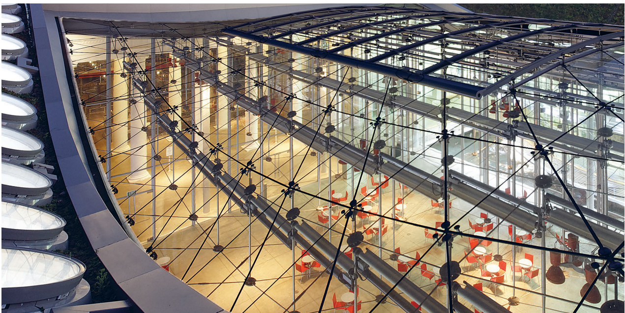
top: California Academy of Science, Exhibition and Research Center, San Francisco, 2008 Architects Renzo Piano Building Workshop; Facade Josef Gartner
