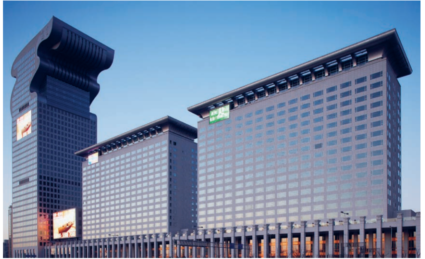
bottom: CNOOC Building, Beijing, 2005 Architects Kohn Pedersen Fox Associates PC; Facade Josef Gartner
